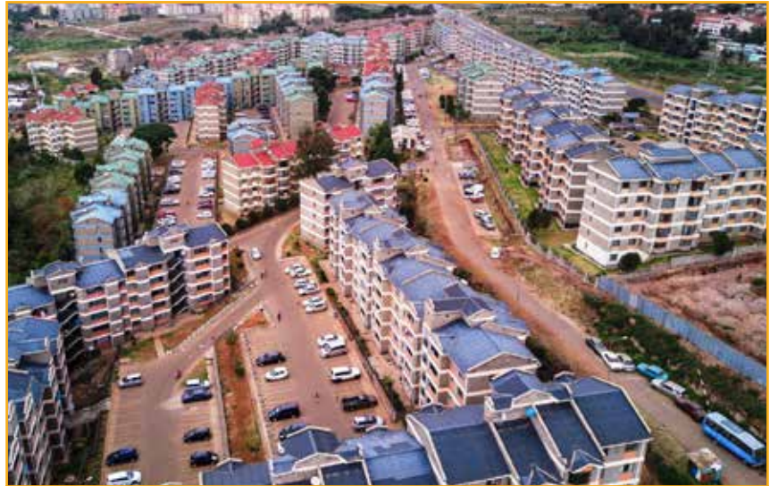
The expansive NHC Langata Estate
