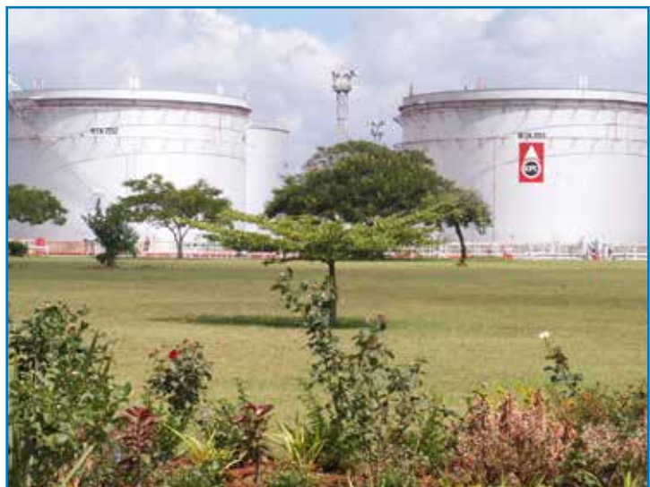
Kenya Pipeline Company storage tanks in Nairobi Terminal.
