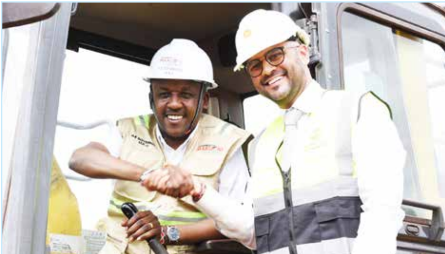
Makueni County Governor, H.E Mutula Kilonzo Jnr and Superior Homes Kenya CEO, Shiv Arora on the excavator during the groundbreaking of a KES. 350 million truckstop at Sultan Hamud. The development is a pilot project of the Northern Corridor Transit and Transport Coordination Authority (NCTCA) implemented by Superior Homes Kenya.
