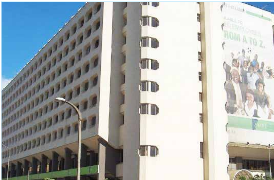
Kencom House in Nairobi's Central Business District.
